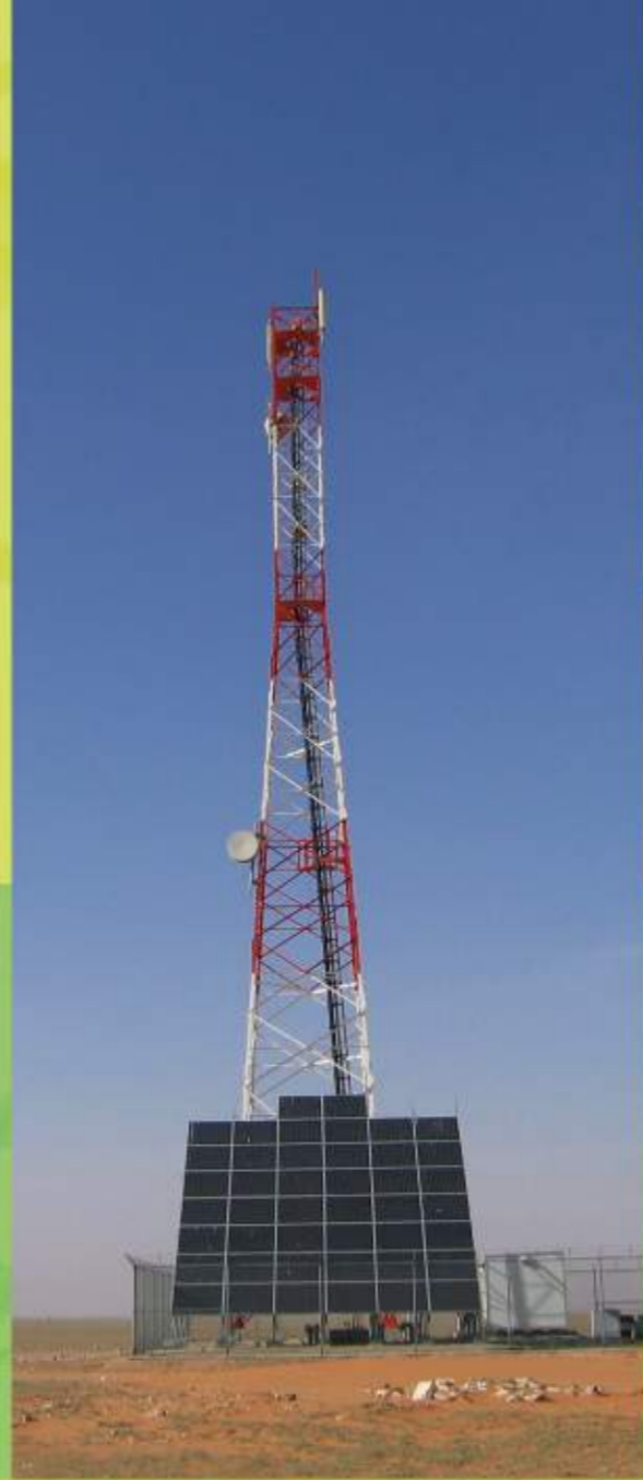
Independent Solar Energy Solution for Railway Communication Station 5-10 kw
