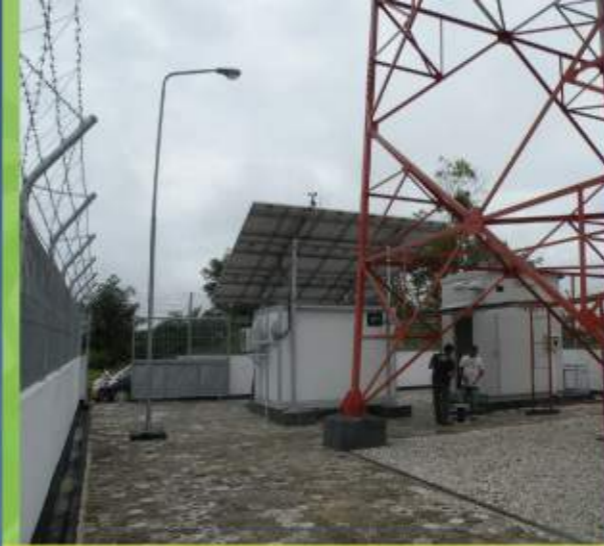
Independent Solar - Wind Energy Solution for Communication Relais Station 1 till 2 kw; 220 V AC / 50 HZ
